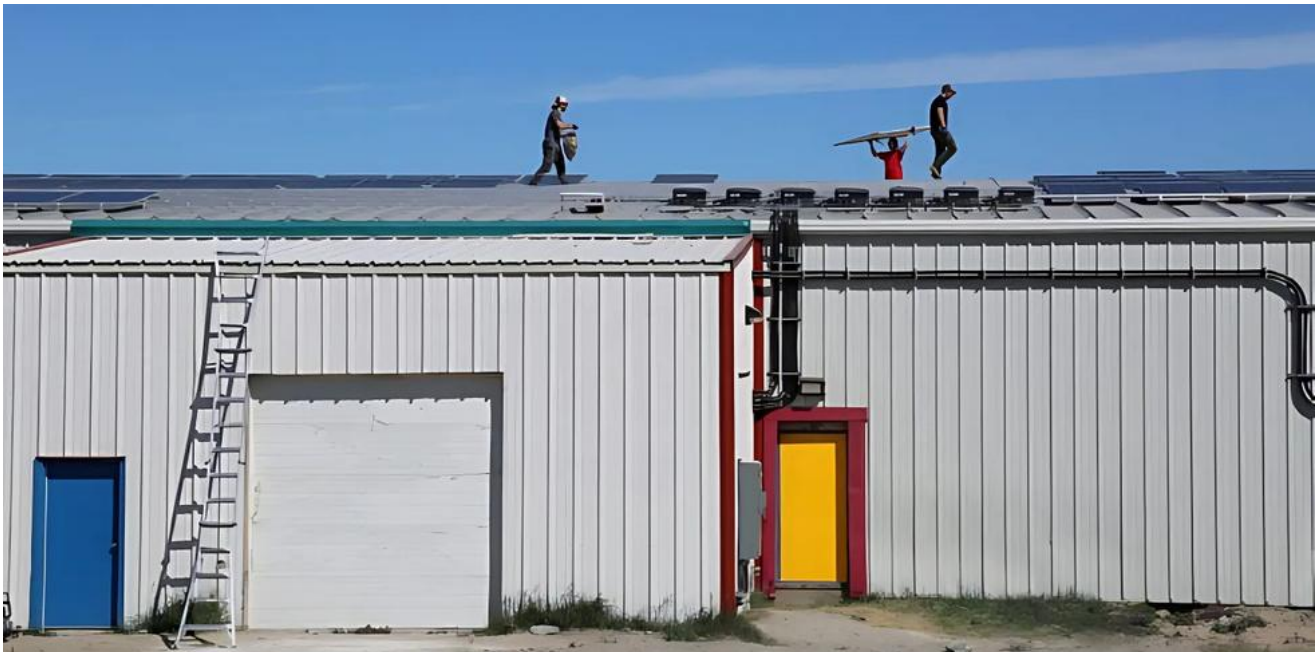
Figure 15: Solar panels being installed on the roof of the Noel Nuvak Arena in Chesterfield Inlet
