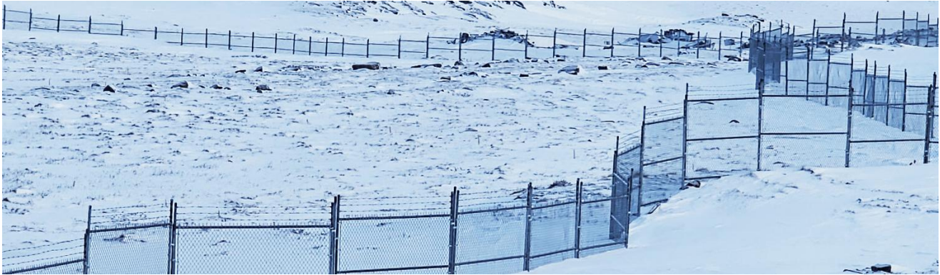
Figure 42: Typical fencing around a large-scale solar array 51
