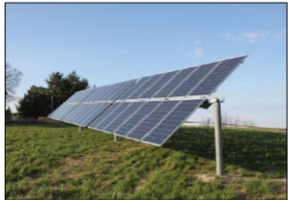
Single Axis Tracker Mounting System
