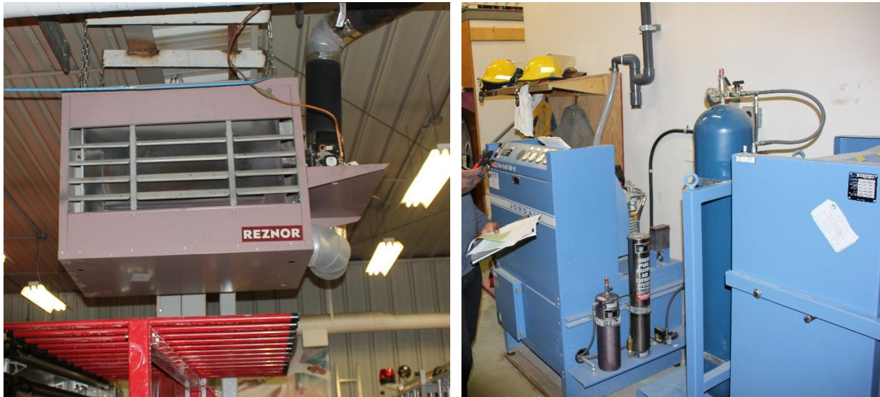
Figure 2: Reznor Unit Heater (left), Jordair Oil Furnaces (right)
