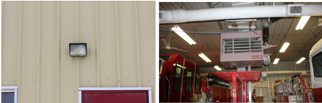
Figure 4: Exterior Wall Pack (left), and Interior Fluorescent (right)
