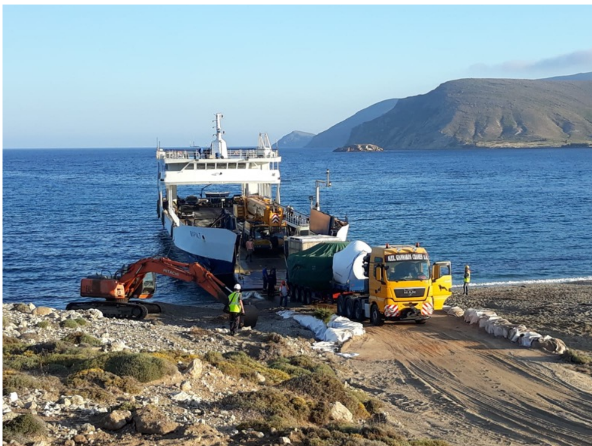
Figure 34: EWT turbine components being transported from barge to beach using a temporary ramp.
