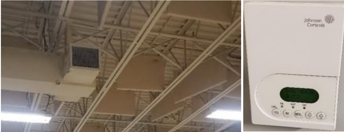
Figure 4: AHU supply duct (left), Johnson Controls Programmable Thermostat (right)
