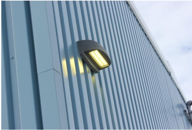
Figure 5: Exterior Wall Pack (left), and Interior Fluorescent (right)
