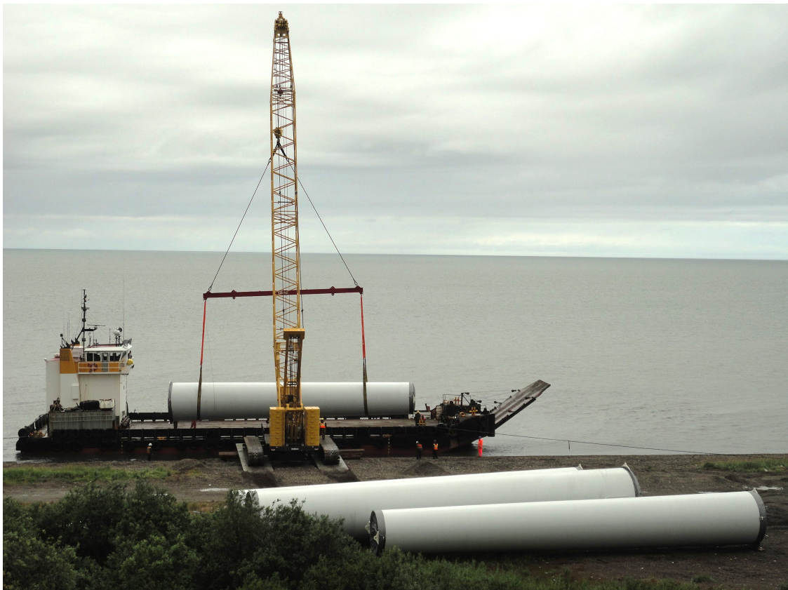
Figure 32: EWT tower sections being lifted from barge to beach using a mobile crane.
