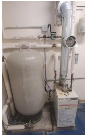
Figure 5: Toyotomi DHW Heater, Expansion Tank and Recirc Pump
