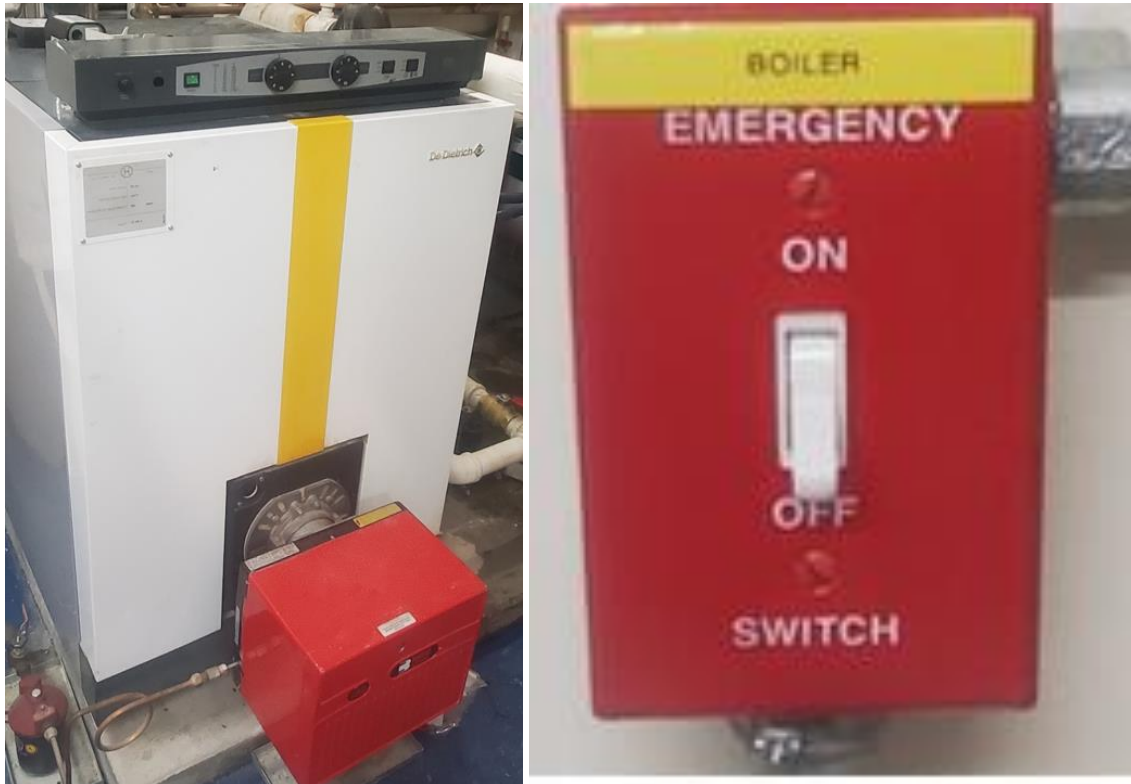
Figure 2: De Dietrich Boiler (left), boiler switch (right)
