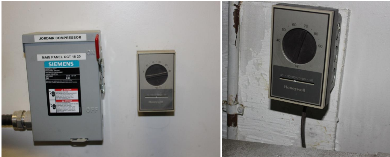
Figure 5: Jordair Oil Furnace Thermostats
