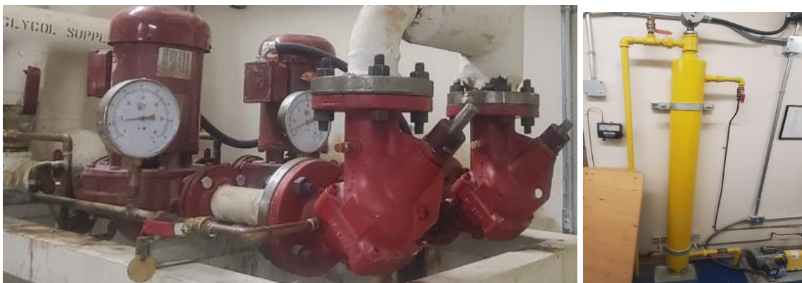
Figure 3: Glycol Circulation Pumps (left), Expanded Fuel Oil and Supply Pump (right)
