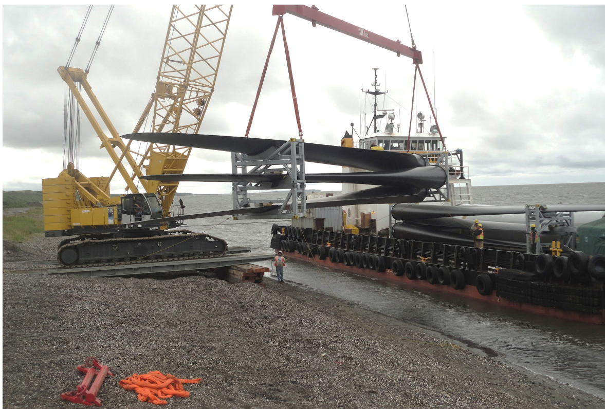
Figure 33: EWT blades being lifted from barge to beach using a mobile crane. Sets of three blades are held in a custom-made cradle for safe transport.
