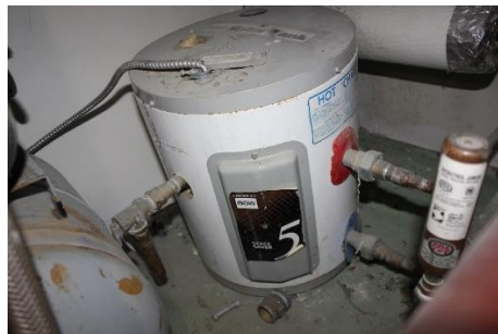
Figure 3: Failed DHW Tank
